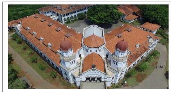
Figure 12. View of the building
